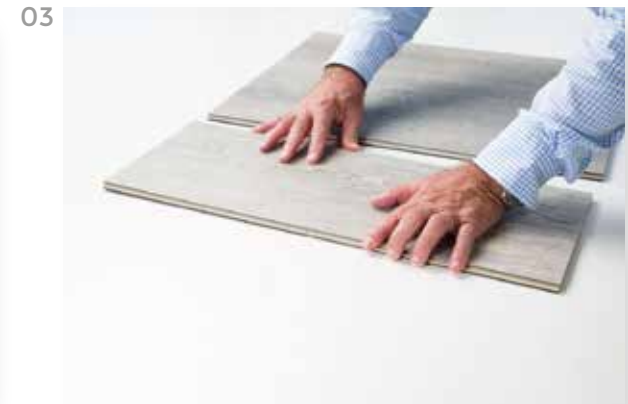
Place the planks gently on the floor
