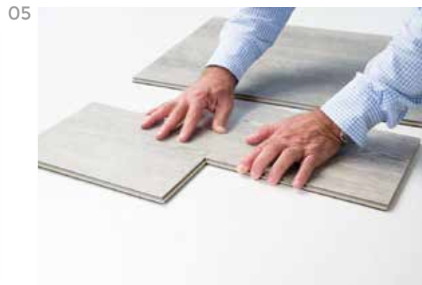
Press the planks gently while sliding
